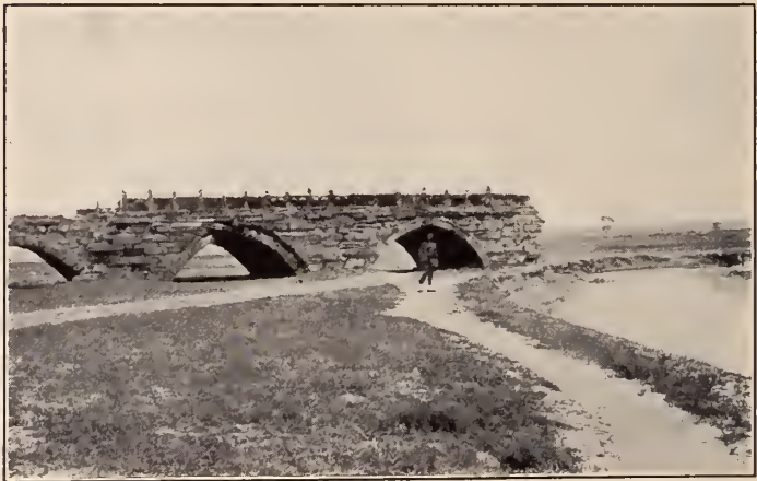
A silted-up bridge in Shansi. One of the ultimate results of deforestation
